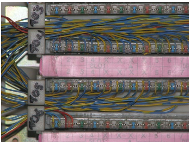
Figure 2 IDC 110 punch block for ethernet installations [Wikipedia]
